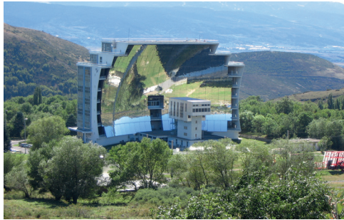
Figure 14. Solar Thermal: Concentrated Solar Power (CSP)
